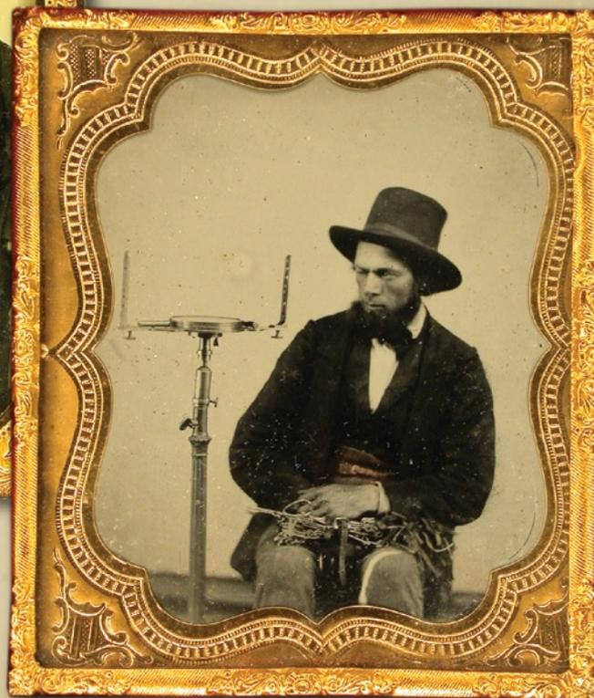
**Plate 5 (right)** As if to take a sight – this surveyor peers through the compass sight vanes (one might wonder if the photographer's assistant isn't lying on the floor out of view to hold the Jacob's staff upright). His measuring chains and pins are across his lap. (Sixth-plate ambrotype) *Author's collection.*
