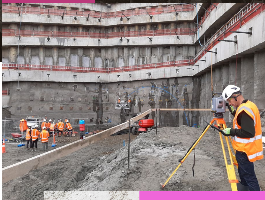
Survey team setting out initial foundation work for tunnel construction.
