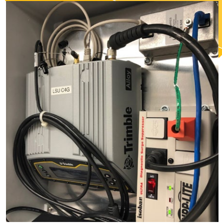
Inside an LSU C4G GNSS base station enclosure that has access to Ethernet and AC power.
