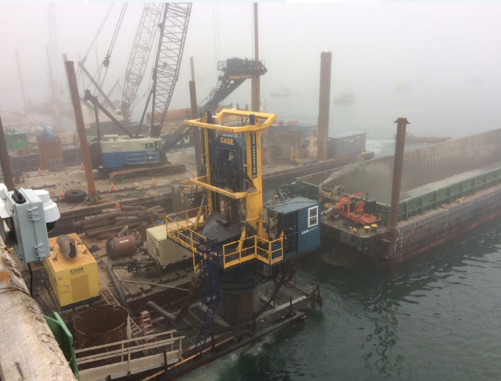
Working with the Eastern Division of Case Foundation, CPM drew upon the benefits of the GNSS solution to help set the piles for the new bridge. The system's ability to function in fog, as shown here, proved huge.
