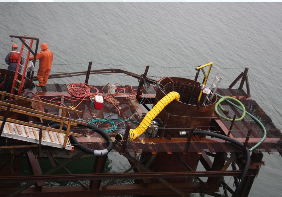
With the drilled shaft cage set in place, latent concrete from the shaft pour is removed in preparation for setting of the column cage itself. There were 14 new caissons installed to support the new piers.
