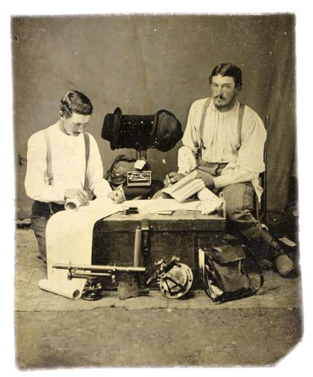
**Plate 7** An incredible tintype taken in the mid-1870s shows an entire inventory of items used in the field. With their hats on the chair back, we see a measuring tape and drafting set on the chair seat. They sit around a camp trunk with maps, ink and field notes on the lid. Before the trunk is a wye level, hatchet, transit and backpack. *Author's collection.*
